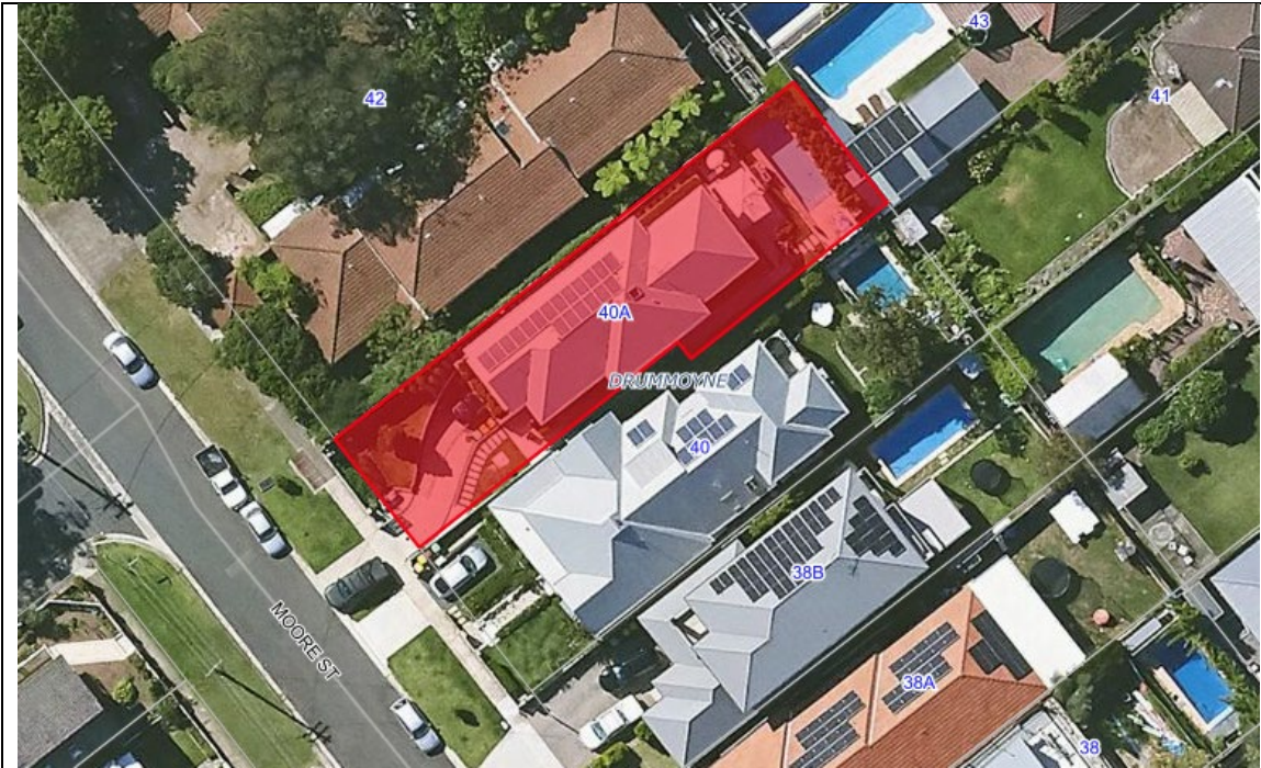
Figure 2. Aerial view of 40A Moore Street, Drummoyne - showing construction of a new dwelling.
